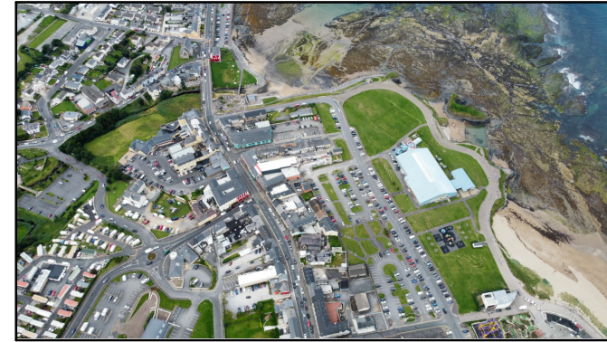
RENNISONS LANE AERIAL IMAGE - 03
