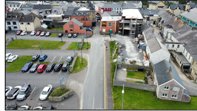
RENNISONS LANE AERIAL IMAGE - 02
